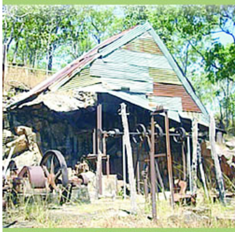
A derelict mining spot in Jos
