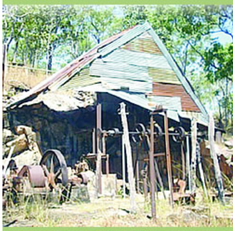
A derelict mining spot in Jos
